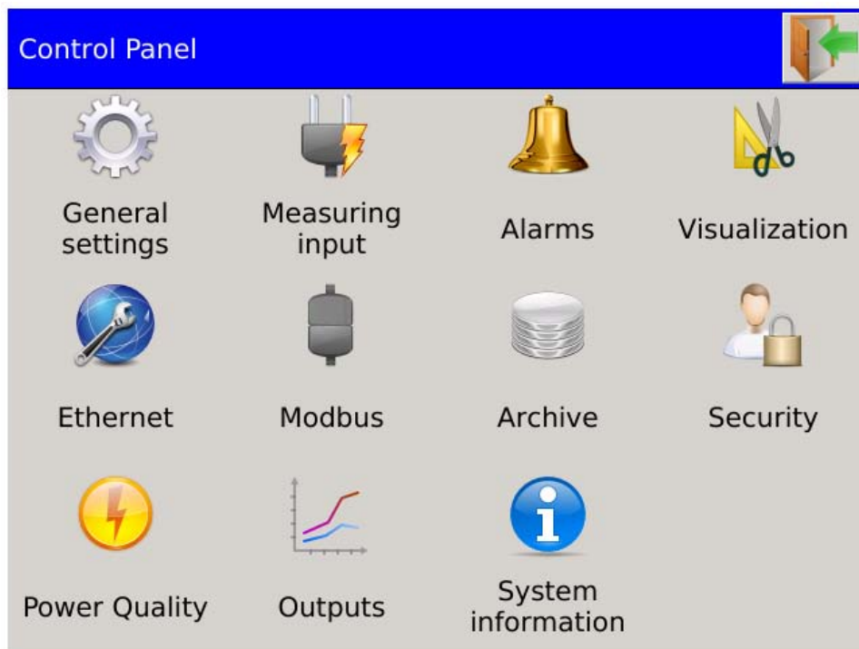
Fig. 36. Control panel - main screen
